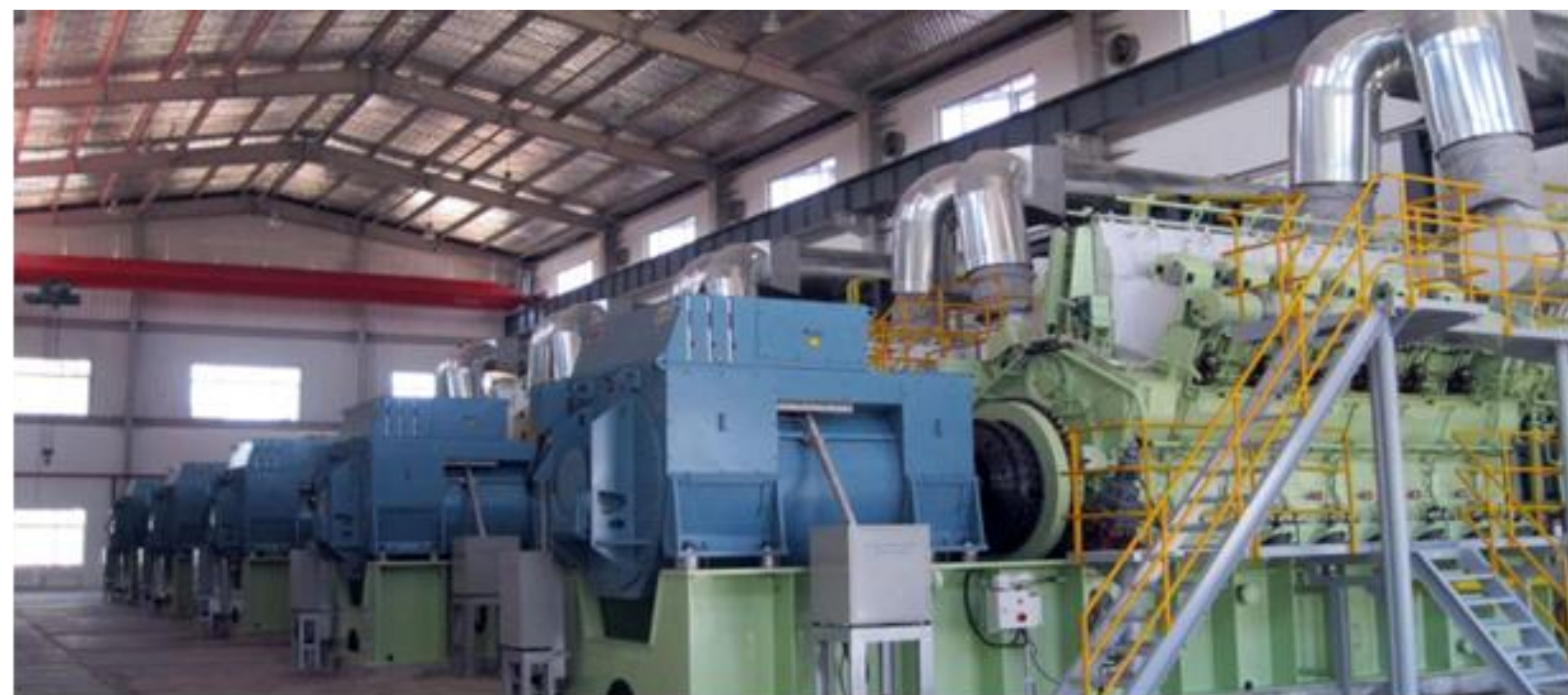
📍 60MW Heavy oil power station project 📅 2010
