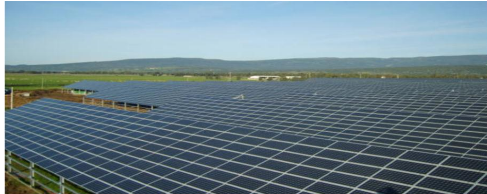
📍 Oristano Province, Italy 📅 2011 🏠 5.9MW
