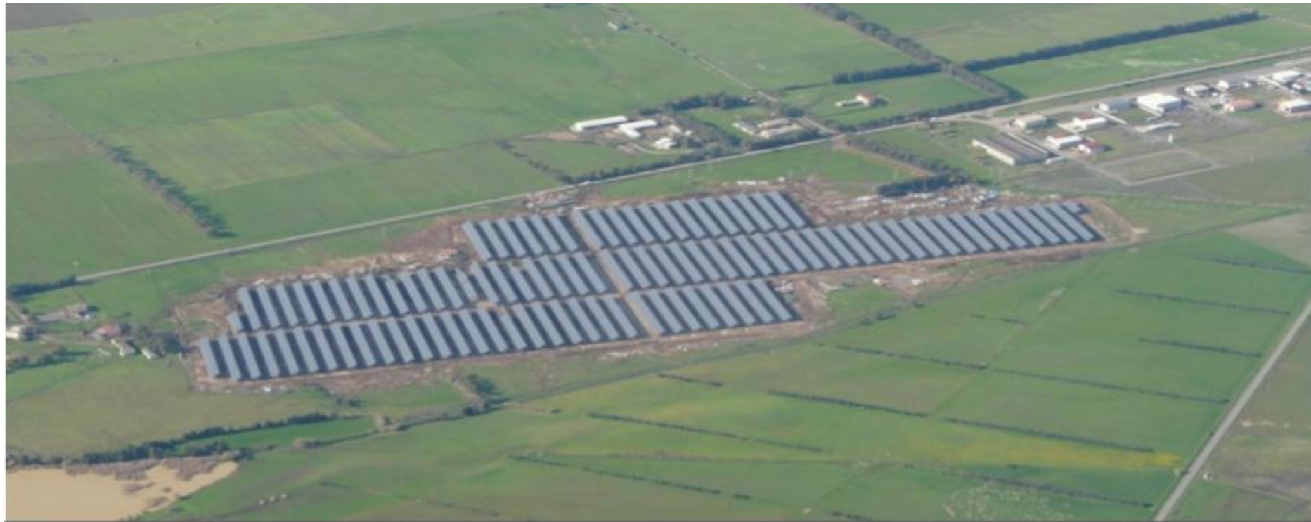
📍 Oristano Province, Italy 📅 2010 🏠 5.9MW
