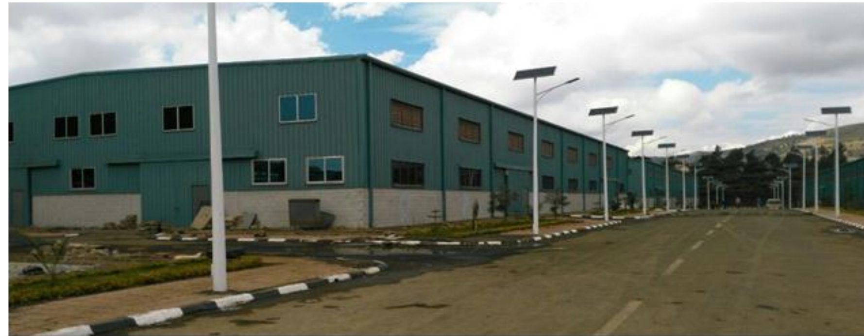
Transformer plant , outer door scene 2015
