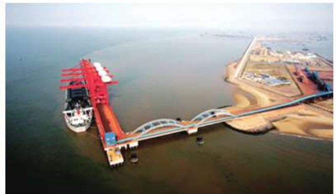
● 矿石码头 Ore terminal
