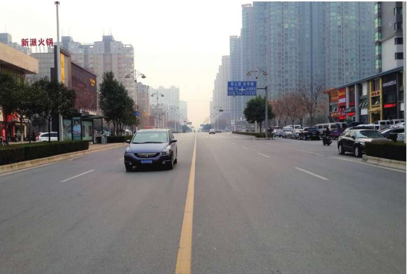
● 长兴街 Changxing road construction work
