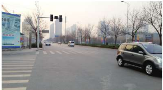
● 洛阳新区展览路工程 Luoyang new town Zhanlan road construction works
