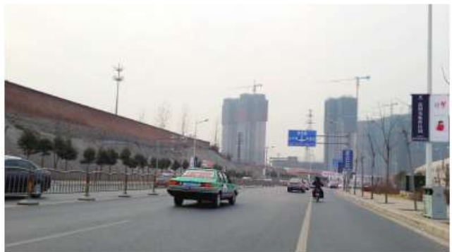
● 洛阳市瀛洲北路 The second phase of Yingzhou north road project
