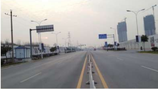
● 洛阳市九都西路 Luoyang Jiudu west road new construction
