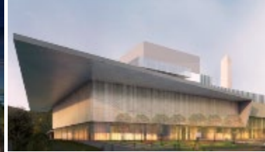
XIAN GAOLING WTE PLANT 3 rd Batch of MoF PPP Demonstration Projects
