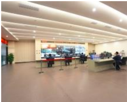
Central Control Room
