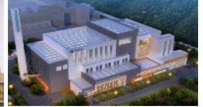
WUZHOU ECO-INDUSTRIAL PARK WTE PLANT 2 nd Batch of NDRC PPP Demonstration Projects
