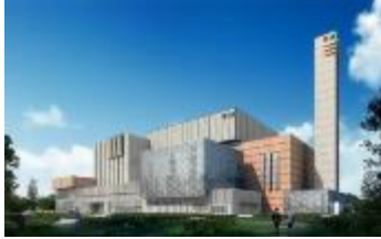
GUANGSHAN WTE PLANT 2 nd Batch of MoF PPP Demonstration Projects
