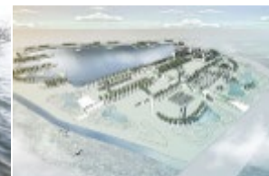
MANAGEMENT OF THE NORTH CANAL IN THE BEIJING, TIANJIN AND HEBEI 2 nd Batch of MoF PPP
