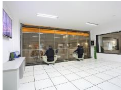
Crane Control Room
