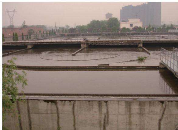
• JiaoZuo City Sewage Treatment Plants
