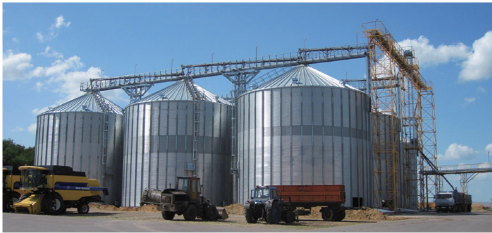
• XinJiang National Grain and Corn Storage Silos
