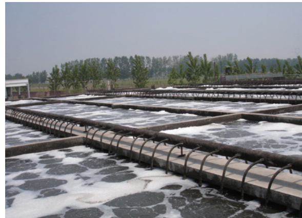
• QinYang City Sewage Treatment Plants
