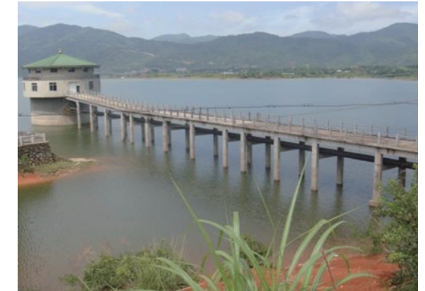
• Construction Site of Water Supply Project for ChangBei International Airport, NanChang
