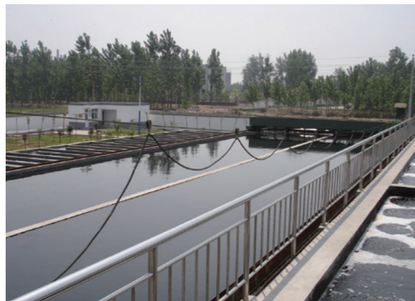
• QinYang City Sewage Treatment Plants
