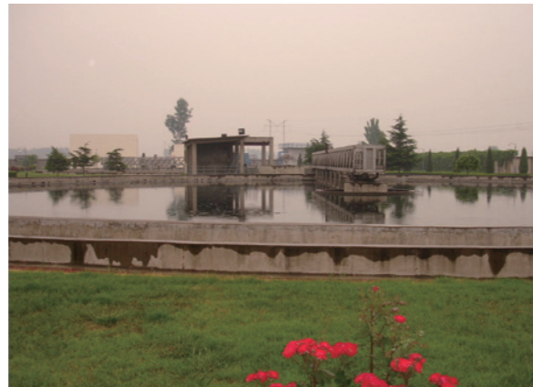
• JiaoZuo City Sewage Treatment Plants
