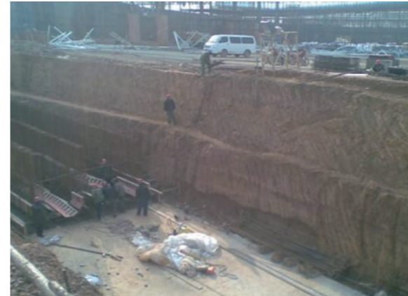
• Construction Site of Water Supply Project for ChangBei International Airport, NanChang
